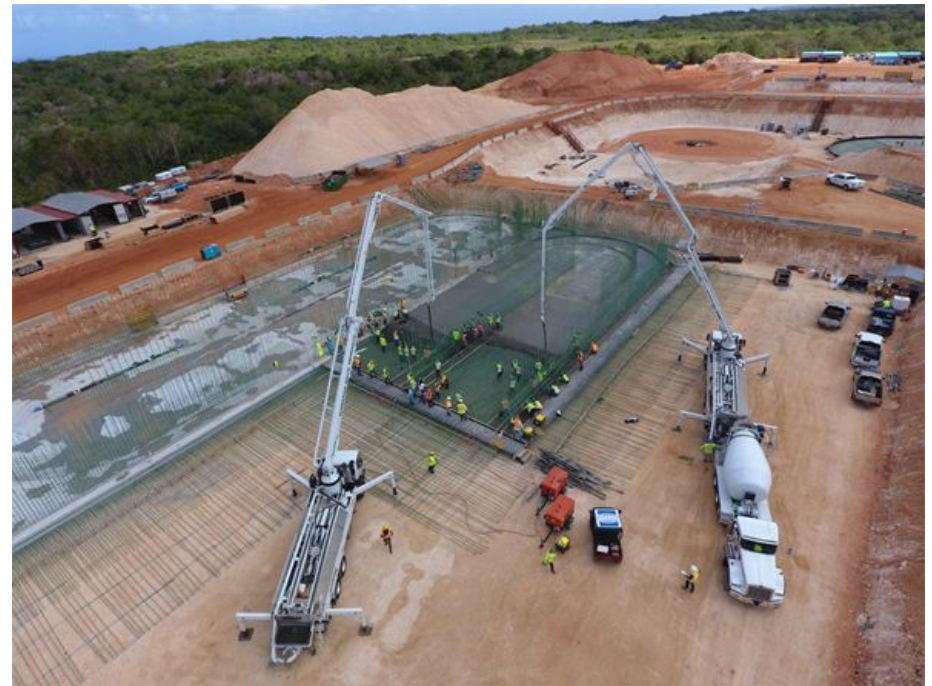
GWA's Critical Infrastructure Projects Continue Black Construction Pouring Oxidation Ditch at NDWWTP
