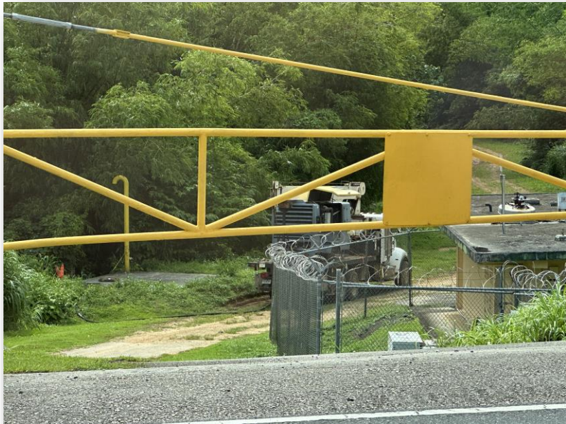
Air compressor set up for NG pipeline pigging
