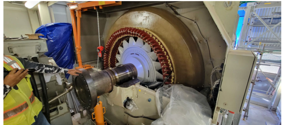
GT#3 Generator rotor coil damage
