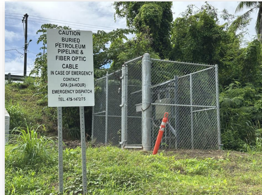
Vegetation management ongoing near pipeline test stations
